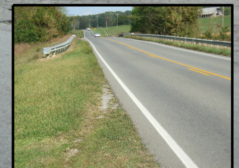
KY 90 Bridge over Glover Creek
